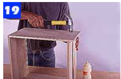
Assemble the drawer box using glue and 6d finishing nails. Note 1/8 x 3/4-in. slots in the drawer sides for hanging-file guides.
