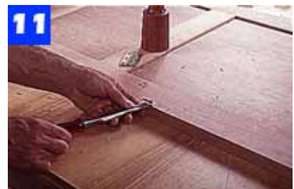
Hold the chisel horizontally to pare away the waste in each hinge mortise. Test the fit of each hinge and adjust as required.
