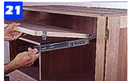
To install the pullout work surface, install support clips on the panel edges and attach the panel to the side-mounted slides.
