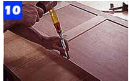
Use a chisel to outline each mortise. Then, make a series of cuts across the grain and about 1/8 in. apart within the waste area.
