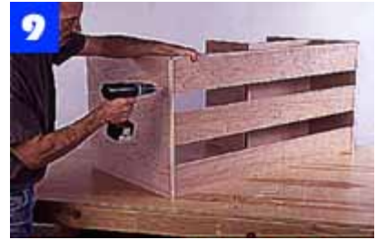
Secure the top stretchers to the lower case sides with screws. Joining plates hold parts in alignment while fastening.
